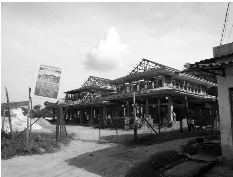
Figure 6. Construction to renovate the Bắc Hà marketplace still underway in August 2008.
